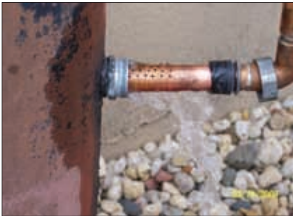
Closeup view of an injection quill.
