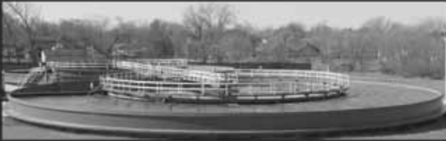
Wastewater Treatment Solutions
