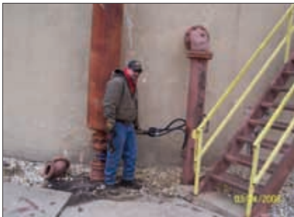
Chad standing between the air header and the Effluent line.
