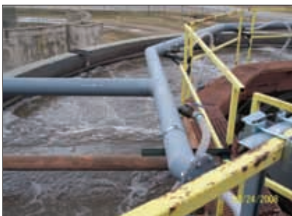
New welded air header with flexible tubing to drop-pipes in the aeration tank.
