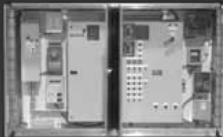
Pad Mounted Control Packages
